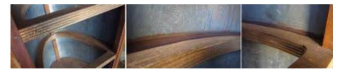
The interior surfaces of lead were then coated with bituminous adhesive sheets of material with silver finish for the specific absorption of vibrations from the speaker. The ribs of the structure were all covered with adhesive strips of closed cell neoprene.
